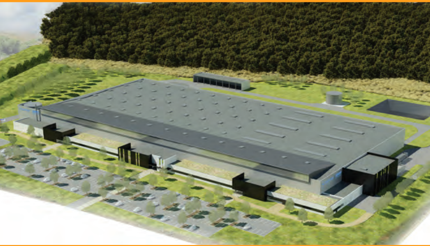
Upper photo: New LEAP production facility under construction in Rochester, New Hampshire. Lower photo: Architects' rendering of new LEAP facility under construction in Commercy, France. Far right photo: An engineer inspects molded fan blade surface during the production process.
